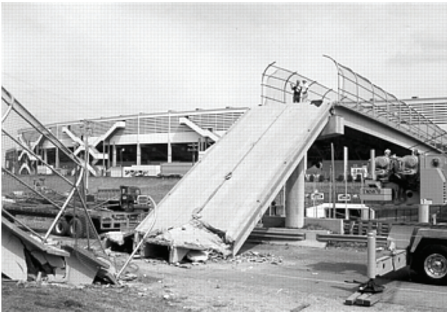
Fig. 2 Collapse of pedestrian bridge over a highway. Source: Ref 1
